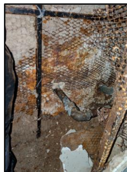
Missing insulation on cold water supply
