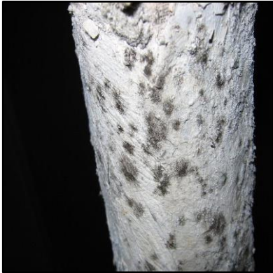
ACM- Pipe insulation (T.S.I)
