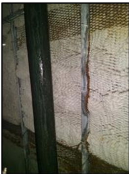
Missing insulation on cold water riser
