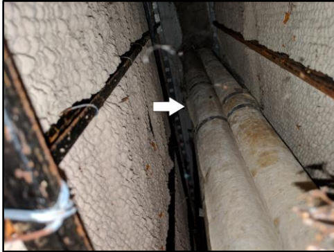
ACM- Pipe insulation (T.S.I)
