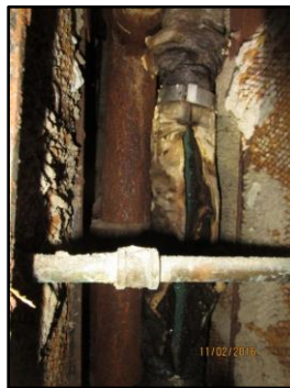
Damaged insulation on cold water riser
